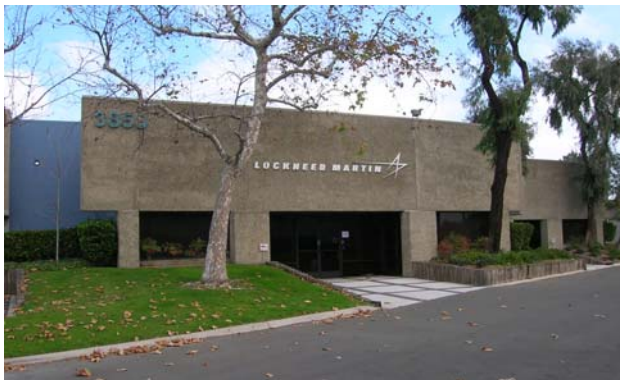
Kearny Mesa Offices
