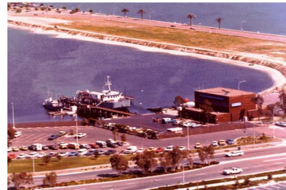
Harbor Island Facility (Circa 1970)
